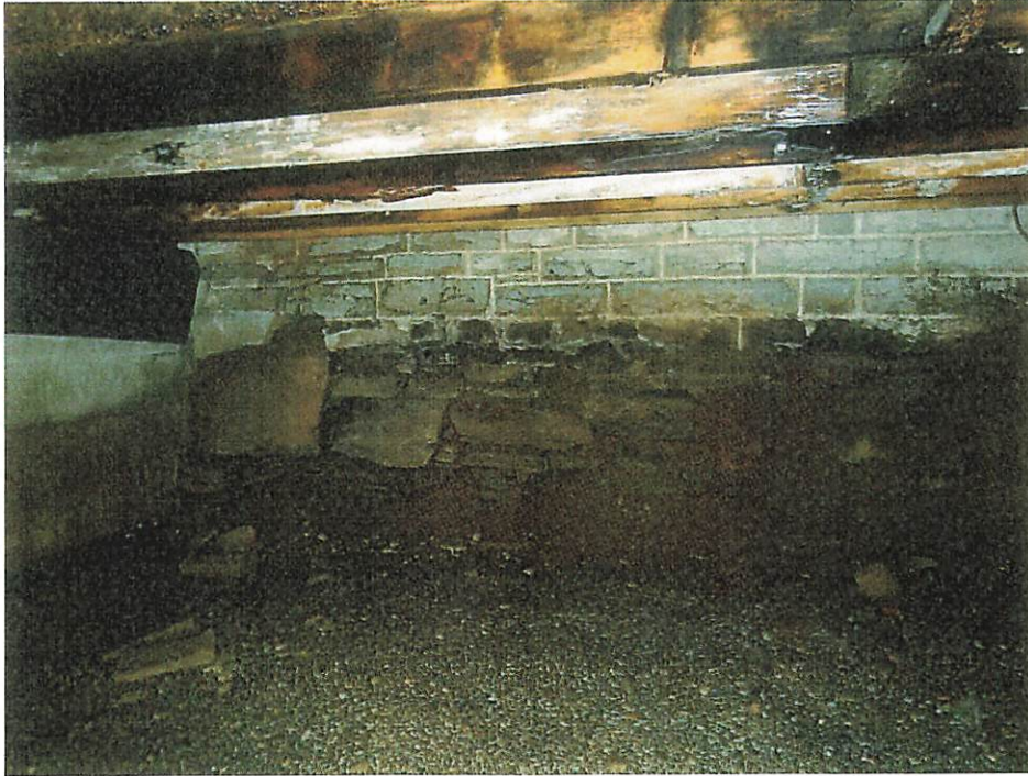
Photo 23. Crawlspace under addition showing connection to original structure
