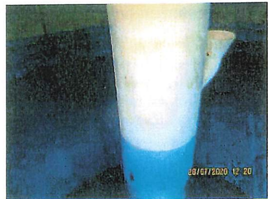
View down at dry riser and overflow from roof
