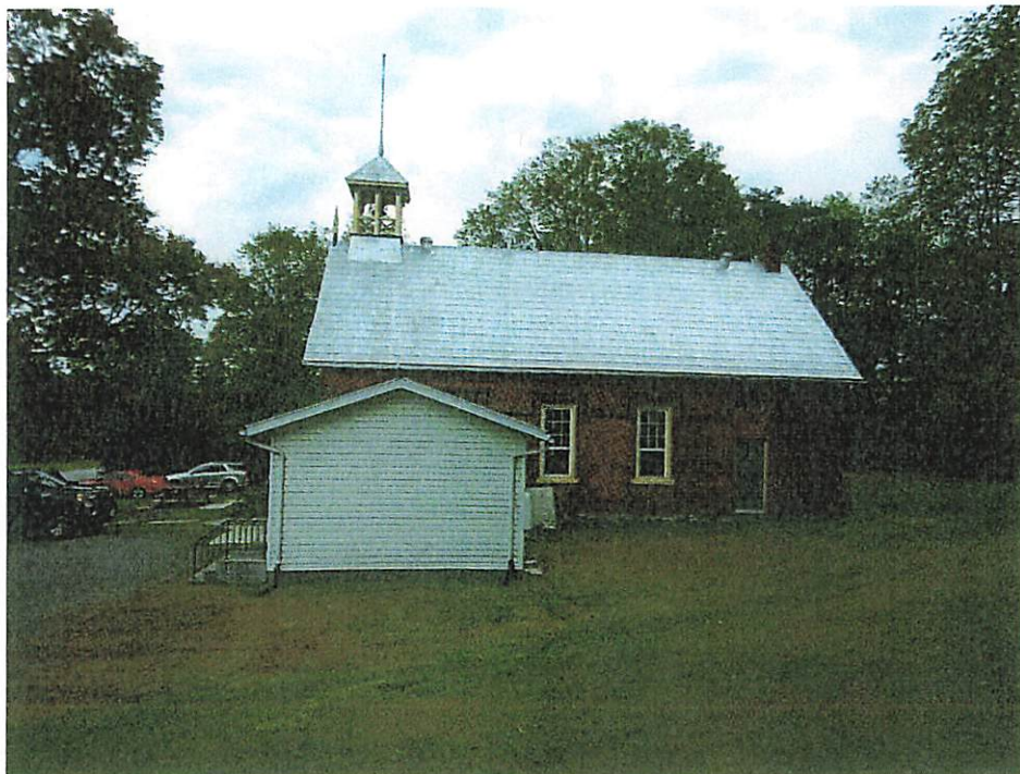
Photo 2. Building west elevation
