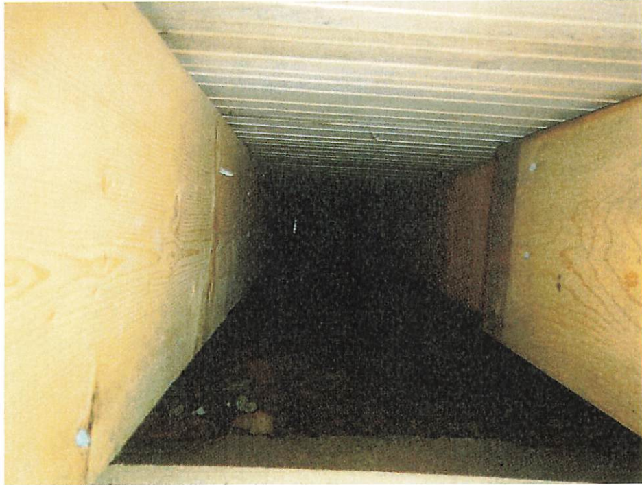
Photo 19. Crawlspace on south side of original building
