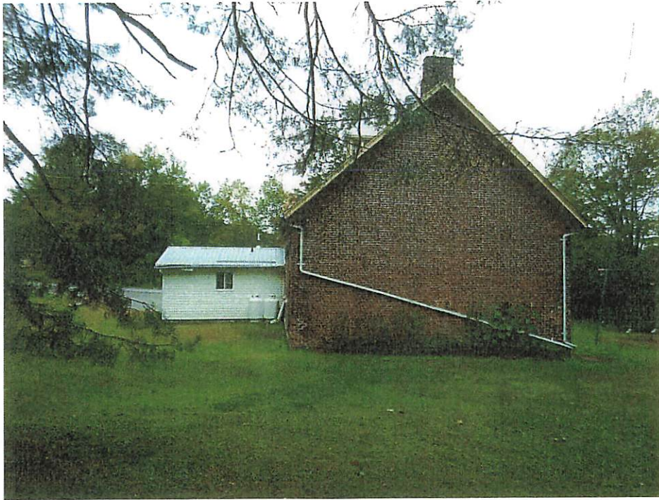
Photo 3. Building south elevation (rear)
