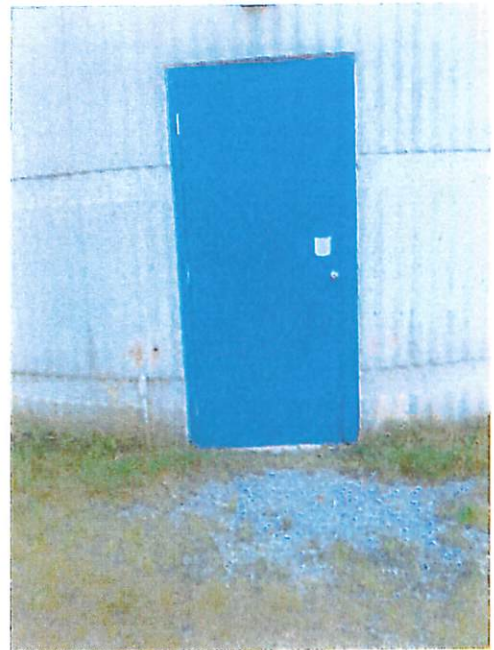
Tower skirt entry door secured after survey
