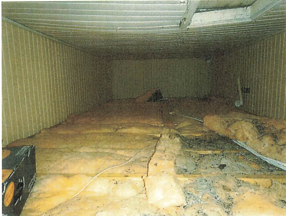
Photo 17. Lower attic space of original building looking west
