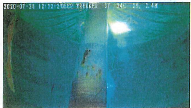
Coating failure at the water level fluctuation zone
