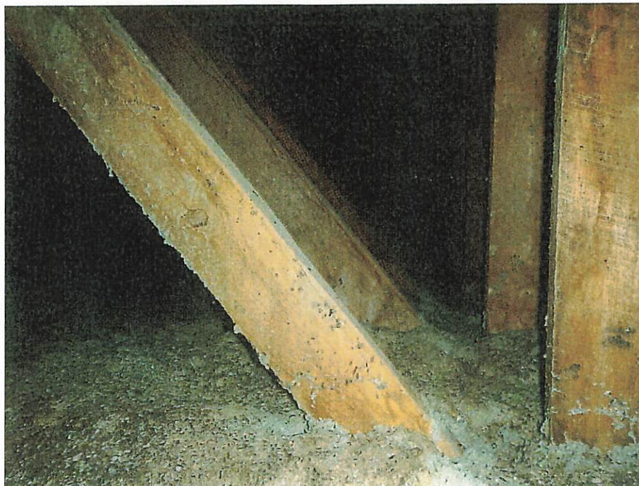
Photo 18. Upper attic space of original building in good condition
