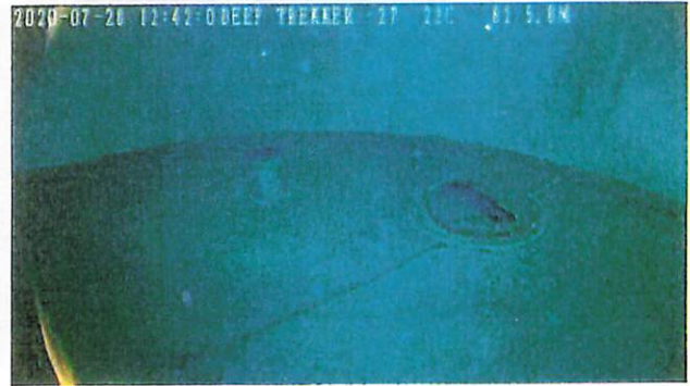
Inlet-outlet pipe, hatch cover, thin sediment layer
