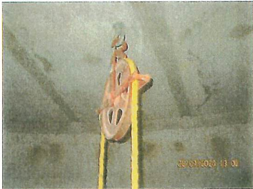
Pulley used for hoisting equipment to tank catwalk
