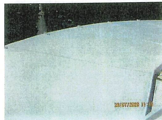
Another random view of tank roof plating
