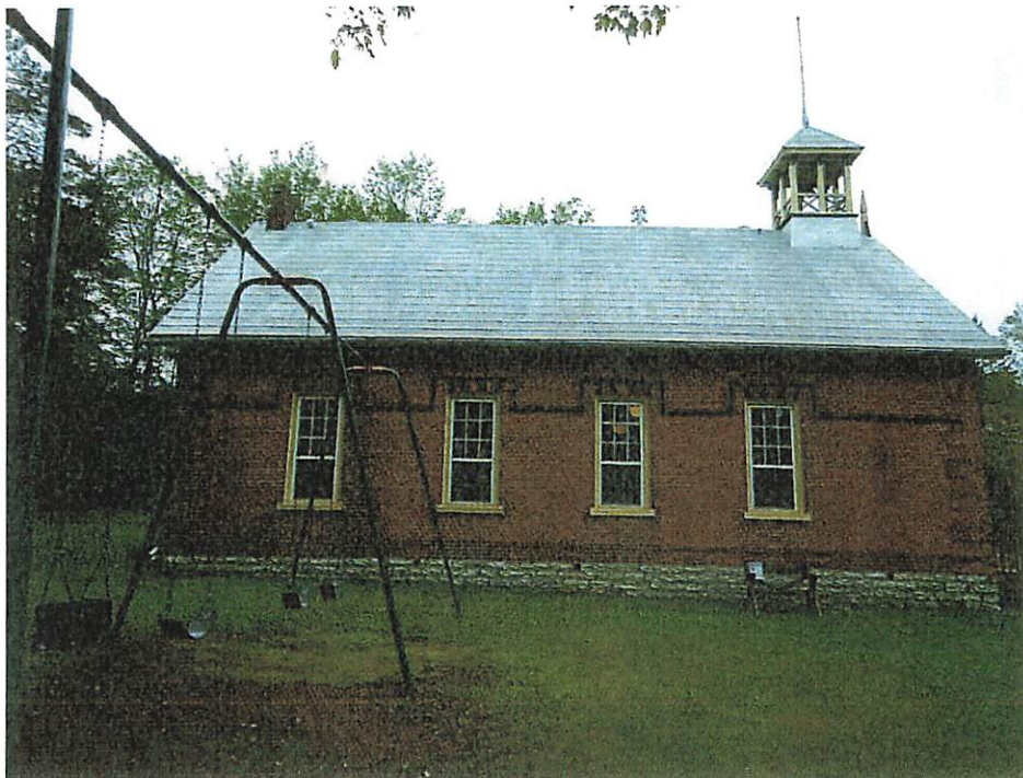
Photo 4. Building east elevation
