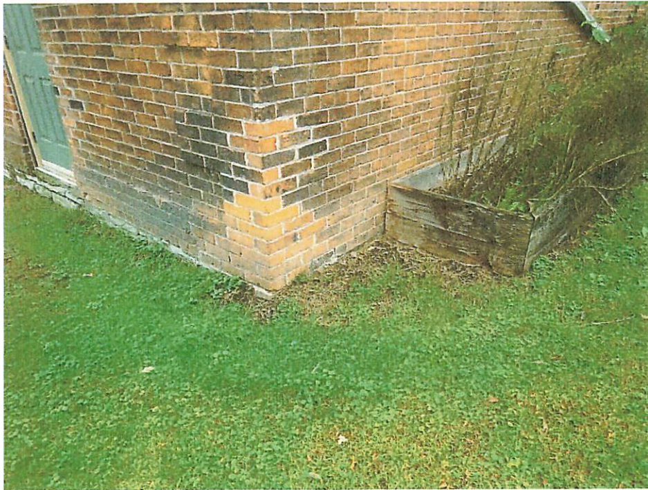
Photo 9. Grading above foundation line
