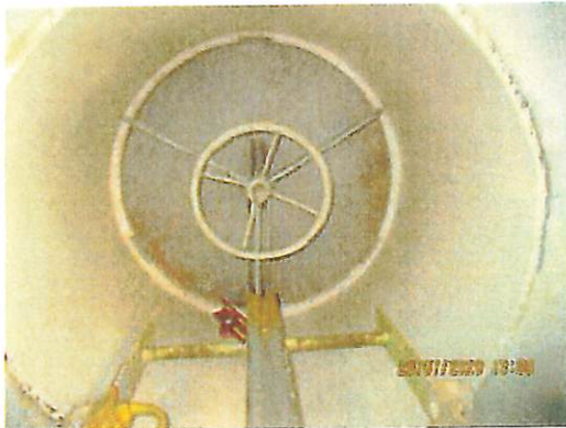
Underside of tank floor hatch
