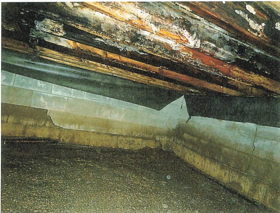
Photo 24. Crawlspace under addition showing condition of floor joists
