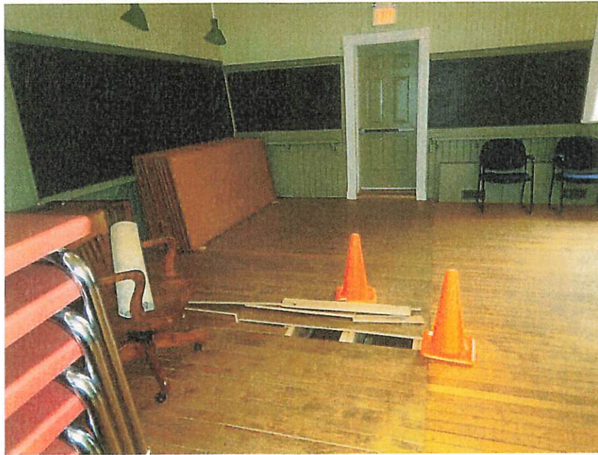
Photo 13. Removed floorboards on south side of building
