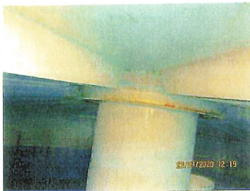
Underside of roof structure viewed from manway
