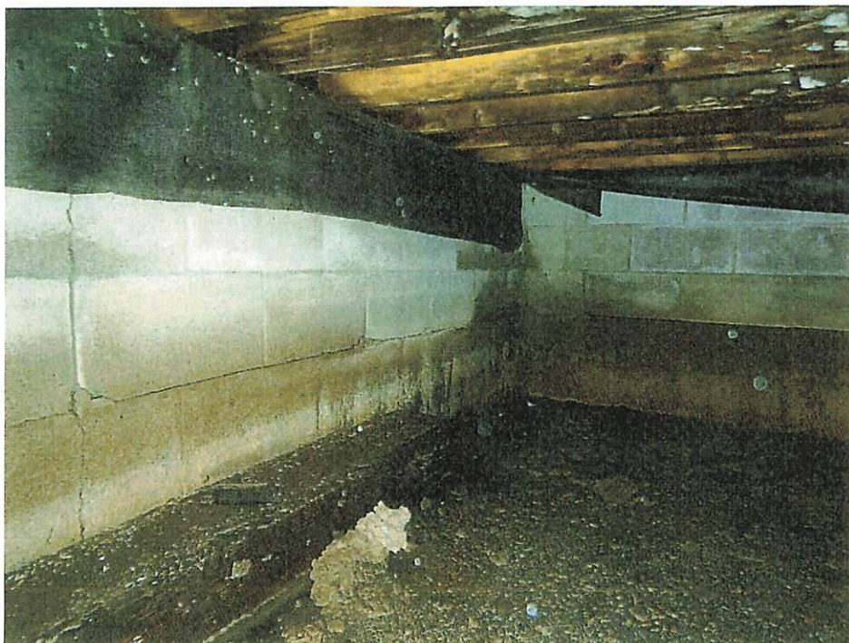
Photo 22. Crawlspace under addition looking west
